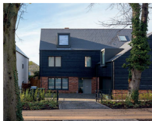
Figure 6.58: On-plot car parking (image above shown space for car parking on driveway and within an integral garage)
