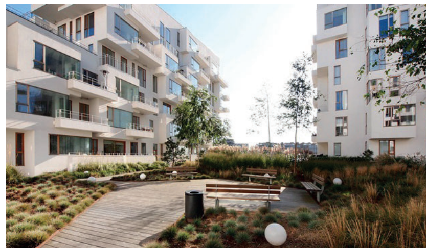
Figure 6.24: The landscape will be drawn into the block, framing views towards the Military Lake.
