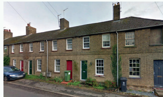
Agricultural brick built cottages in Westwick
