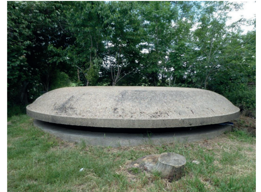
Figure 4.8: This photo shows one of the Oakington pillboxes found within Northstowe. These are to be retained within the Phase 3A proposals.
