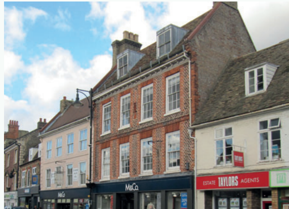
Figure 4.32: Although the building scales and materials vary, the proportions in St Ives Town Centre are similar with a strong vertical rhythm and window proportions consistent across building types.
