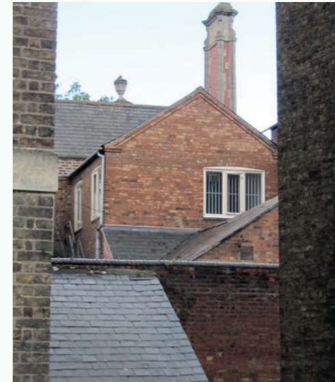
Figure 4.38: The bringing together of a series of simple roof forms creates a rich townscape in Peterborough. Built forms do not need to be complex to be interesting - it is the way that simple forms come together that creates richness
