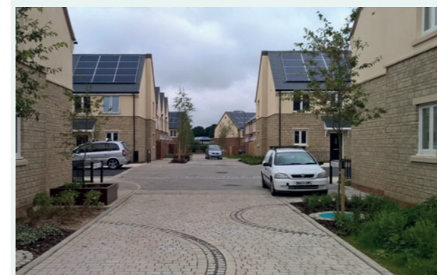
Figure 6.34: Car parking incorporated into the shared surfacing of quieter residential roads.
