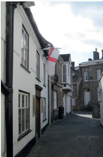
Figure 4.29: Away from the Huntingdon Town Centre, buildings become more informal with varied proportions and sometimes horizontal window proportions
