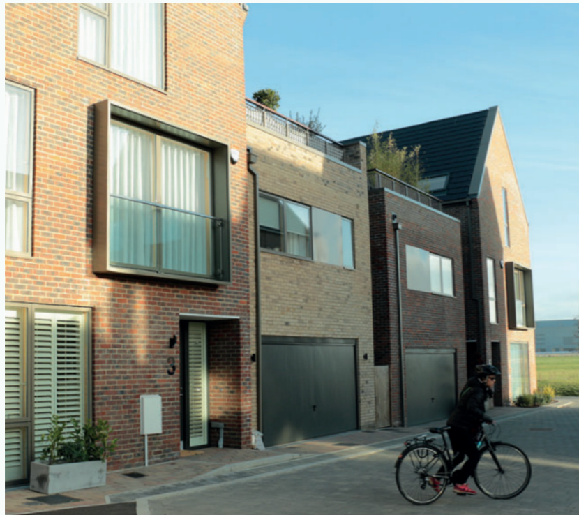
Figure 4.19: Variation in material in this street in Great Kneighton is unified by the symmetrical buildings form, creating a high quality appearance.
