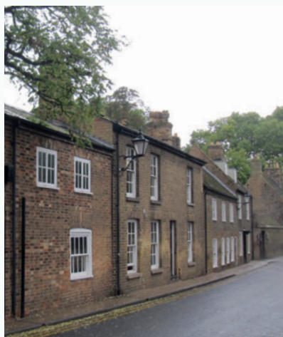
Figure 4.20: Consistent use of a single brick type in Ely brings together these varied building forms.
