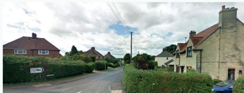
Two storey dwellings set back from the pavement edge characterise much of Longstanton.
