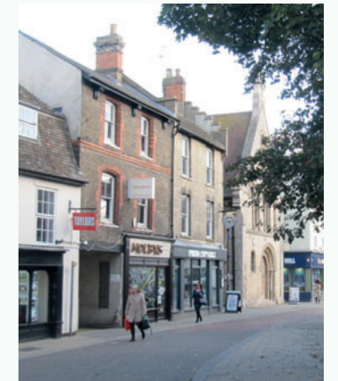
Figure 4.18: Materials vary in Huntingdon Town Centre, but the variety is controlled by being within a limited palette of brick types and render, and varying only building-by-building, not within each building.
