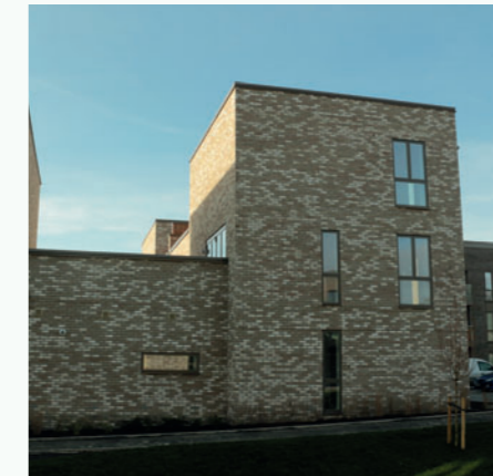
Figure 4.17: Consistent brick used for boundary walls and buildings create a coherent townscape in Addenbrooke's/Ninewells.
