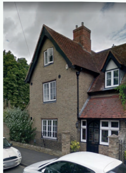
The more historic buildings within the village have a stronger relationship with the street afforded by their minimal set back and visually permeable boundary treatments.
